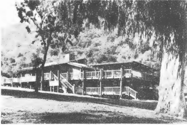
Figure 3.25. This wood structure successfully uses the same material throughout the building—foundation, structure, treatment of railings, wall, and roof material, as well as connection and anchorage details. The design honestly expresses the structure, foundations and other building elements. While it is obvious this is an elevated structure, it still feels very much a part of the site. The foundation members are also integrated well with the building itself (see also Figures 3.54 to 3.57).
